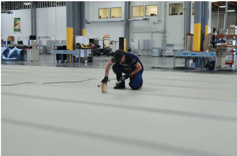
FIGURE 11 Factory fabrication of CSPE panels in Lakeside, Calif. plant
