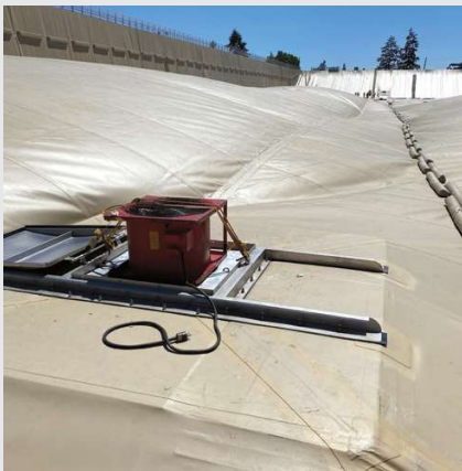
FIGURES 8–9 Inflation via access hatch and west cell cover undergoing inflation inspection
