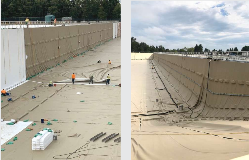
FIGURES 2–3 Installation underway of double trough system on 28-foot divider wall
