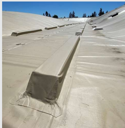
FIGURES 8–9 Inflation via access hatch and west cell cover undergoing inflation inspection
