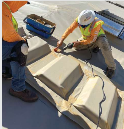
FIGURES 6–7 Crews installing fabricated entry stairways and welding floating cover seams
