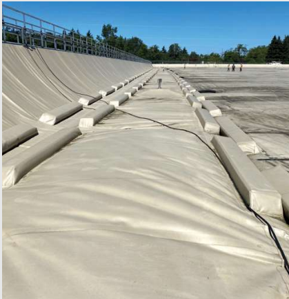
FIGURE 5 Rainwater removal system
