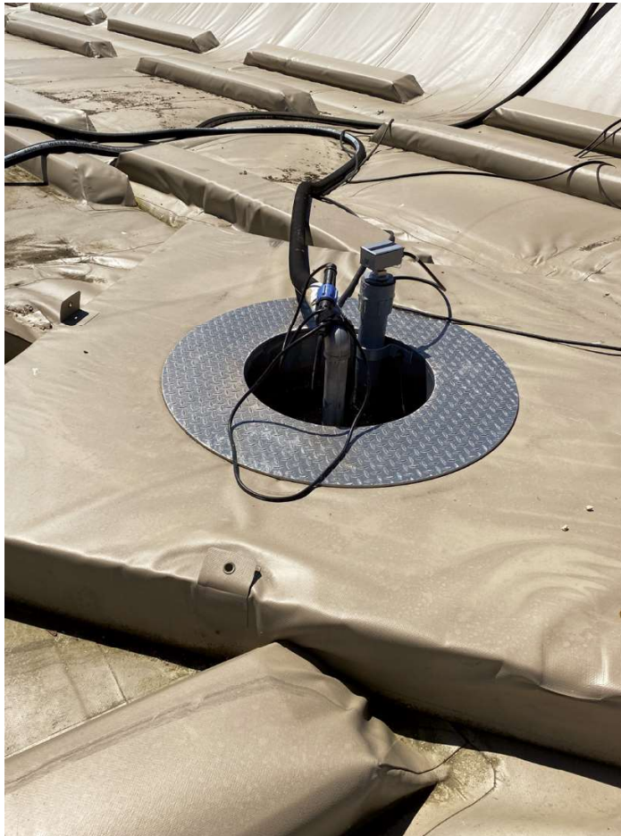
FIGURE 4 East cell divider wall trough in full service
