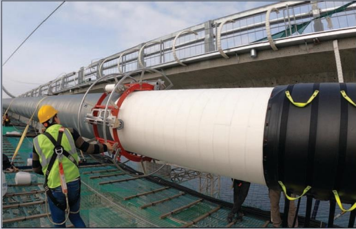
Cableguard is part of the dehumidification system on 1915 Canakkale Bridge.
