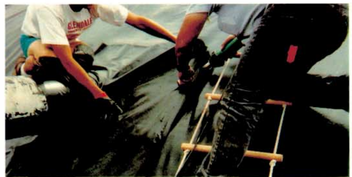
Field seaming during pond construction
